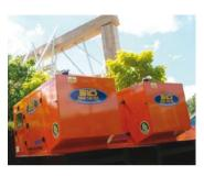
All generators are set to run at 50hz (1500rpm) and can also be set at 60hz (1800rpm).
